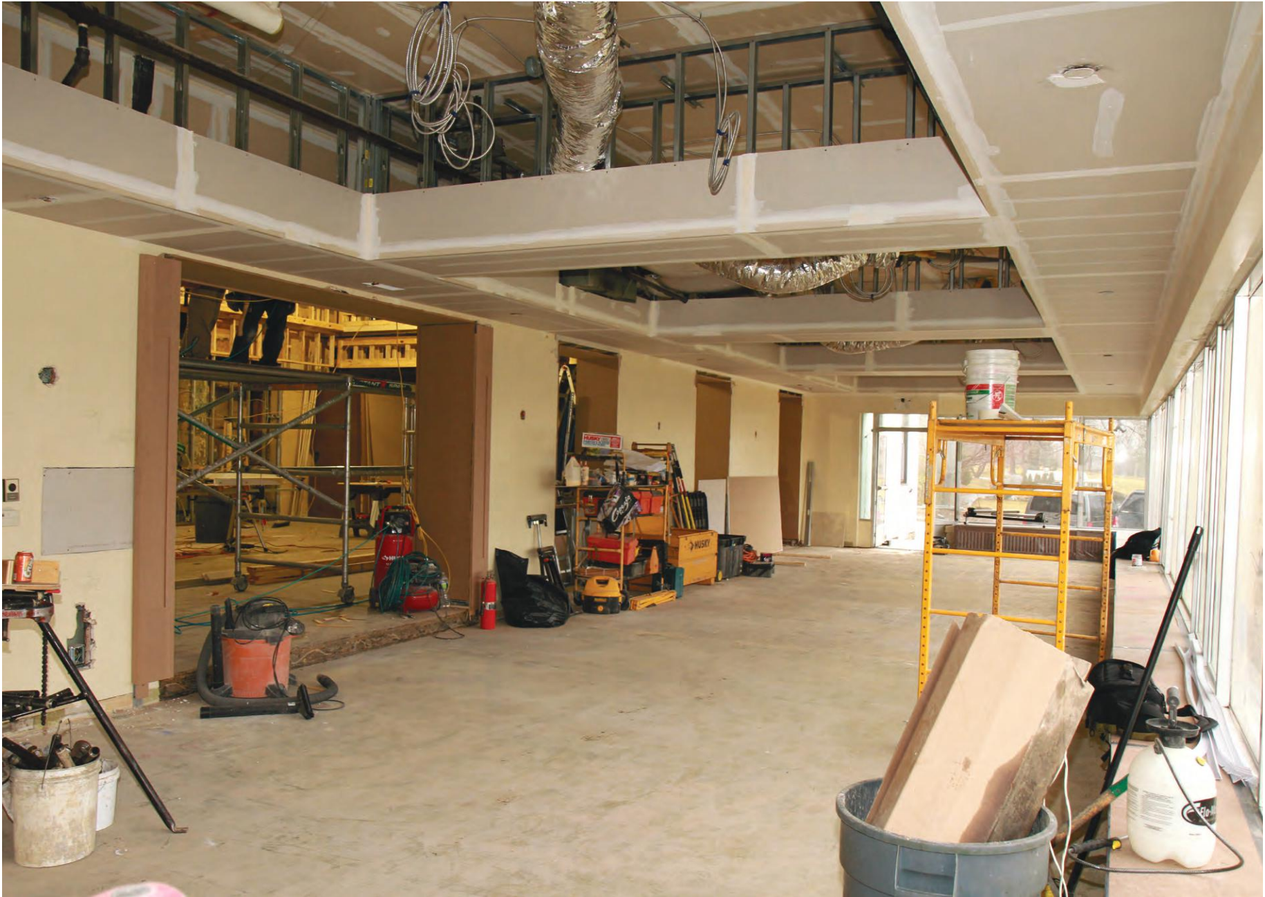
Terrace Room ceiling opened, awaiting new electrical and air conditioning
