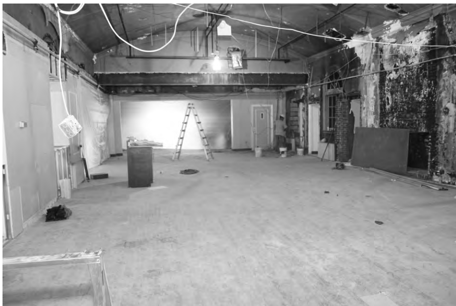
Grand Room immediately after the drop ceiling was removed
